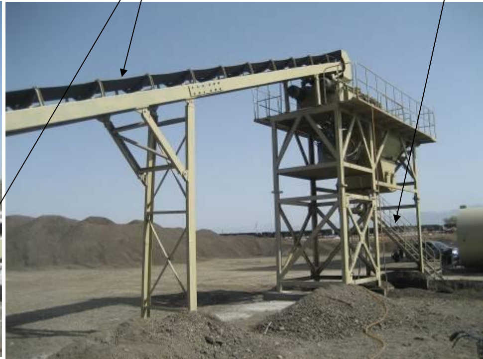
Secondary pugmill (Emulsion Addition)
